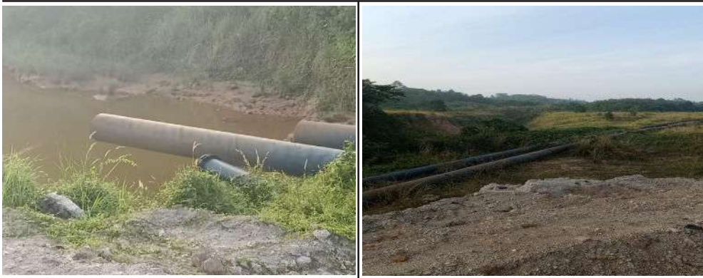
Figure 12. The manipulation of Penimur River Flow using pump
