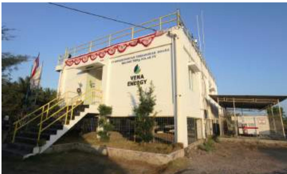
Image 3.1. Selong Solar Power Plant in Geres Village
