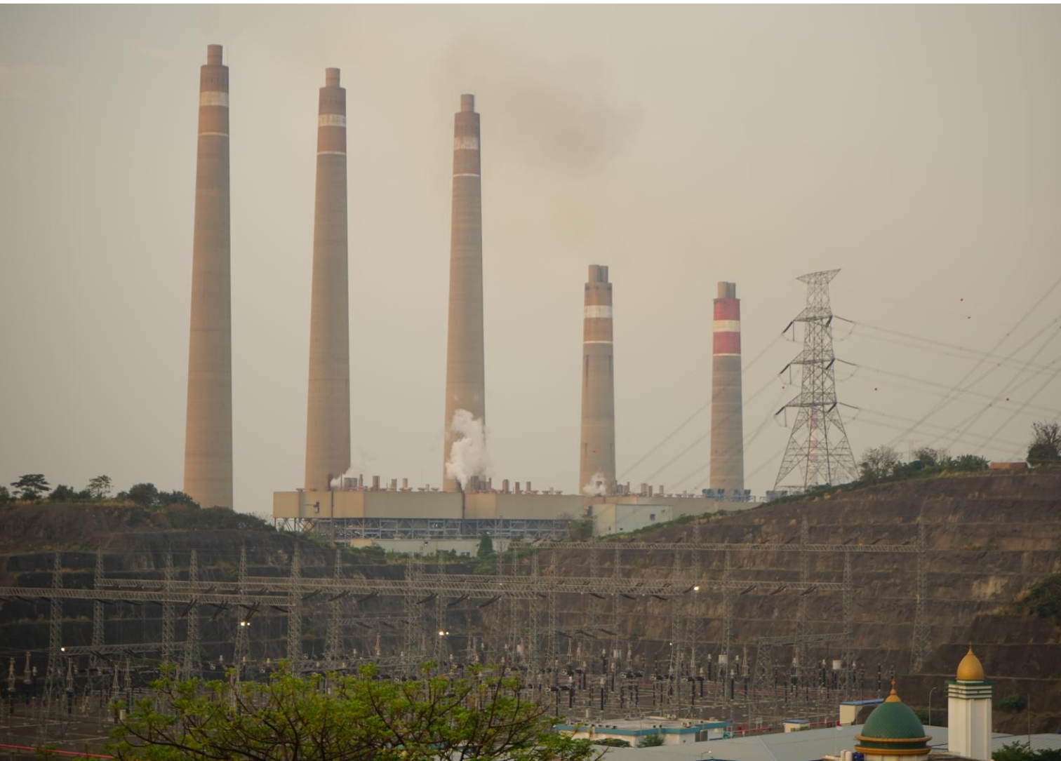
Figure 1. Suralaya Steam Power Plant in Merak, Banten Primarily Fueled by Coal as One of the Energy Resources for the Steel Industry in Cilegon
